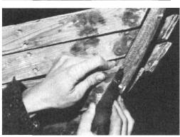
The use of thickened epoxy shows clearly in this photo. It gives the planking a new lease on life and allows these full-length cedar planks, even though slightly damaged and worn, to be used again. For a good fit the second time around, some of the plank ends are dressed down with a block plane, as shown.
