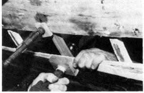
As with the burr setting, the rivet head has to be bucked up on the outside while the riveting takes place. The tool for the job is a heavy iron weight whose end has been shaped to fit into the counterbore and against the rivet head. Steve uses a wooden block on this bucking iron to keep it from sinking the rivet head too deeply in the soft cedar.
