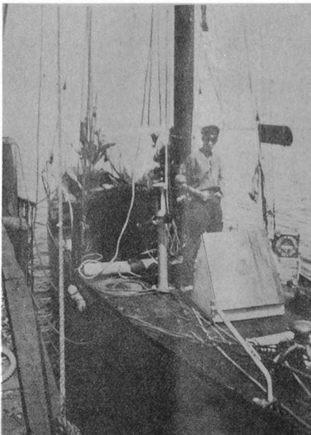
The forward deck, showing hood for forward hatch to keep out water
